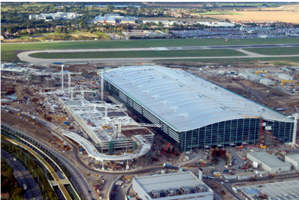
Exhibit 4 – T5 under construction, September 2005
