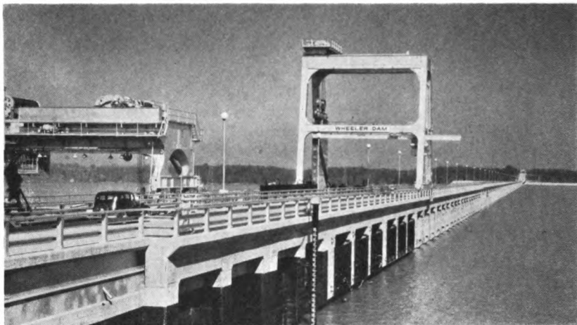
FIGURE 35.—85-ton gantry crane for intake gates.
