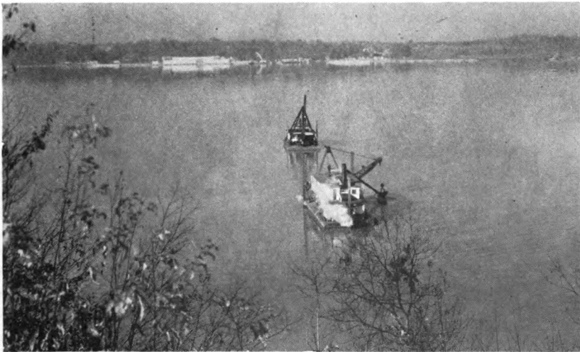
FIGURE 3.— Wheeler site before the start of TVA construction.
