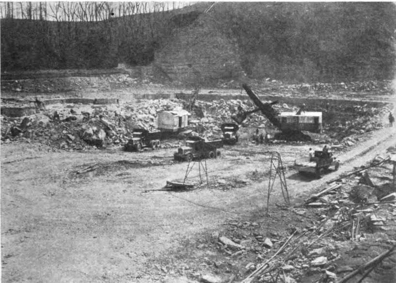
FIGURE 70.—Shovels for foundation excavation.
