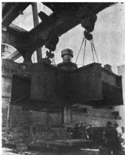
FIGURE 107.—Lower bracket and shaft assembly.
