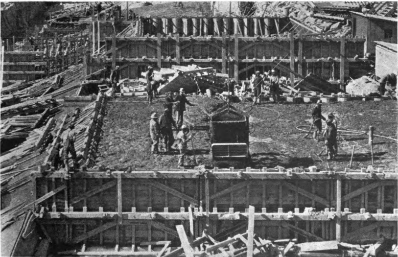
FIGURE 94.—Placing mass concrete.
