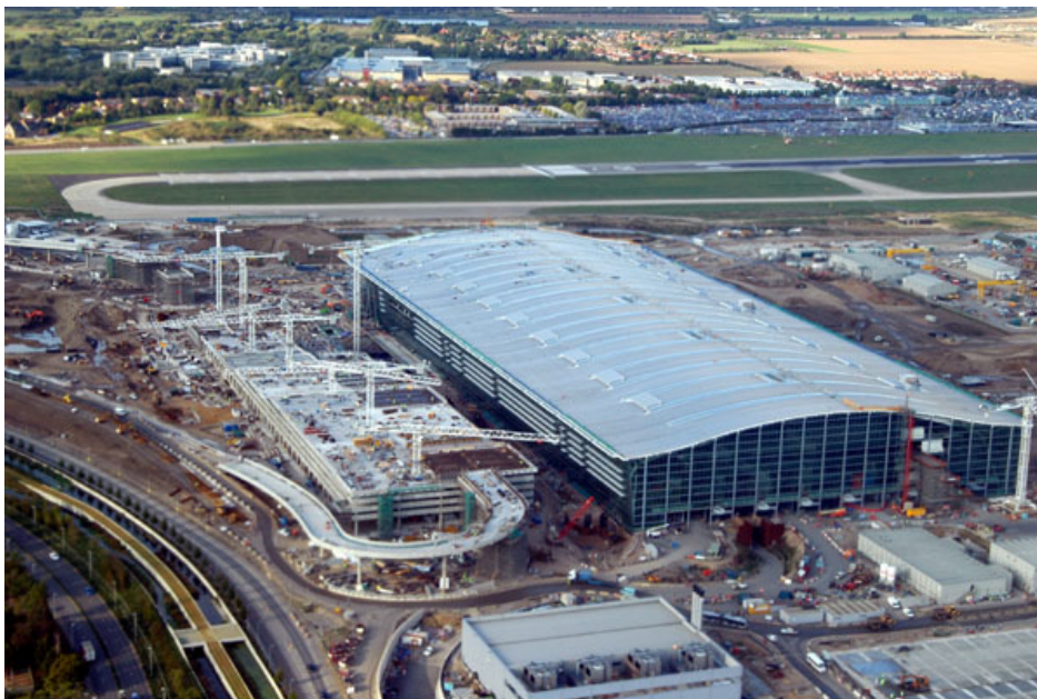
T5 under construction, September 2005
